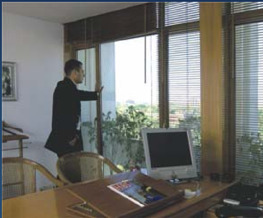
Fenesta windows in office room
